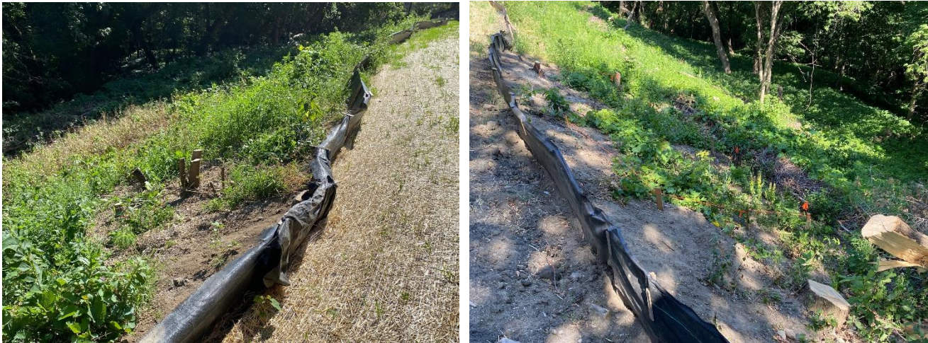
FIGURE 2. Aug 01, 2022. East Test Area (left). West Test Area (Right) After staking out locations & Before weeding, terracing, seeding, covering with erosion blankets & planting plugs.
