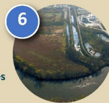
6 Cargill East River Dredge Site Culvert (see page 8)
