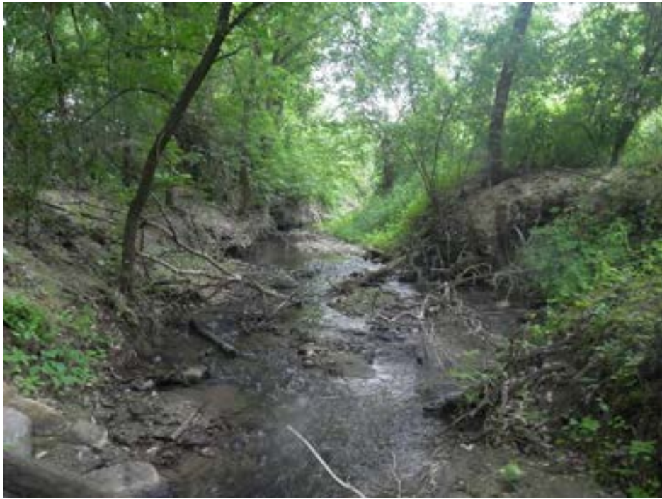
Photo 26. LMRWD Reach. Channel degradation and bank erosion (looking upstream). A scarp can be seen on the right side of the picture
