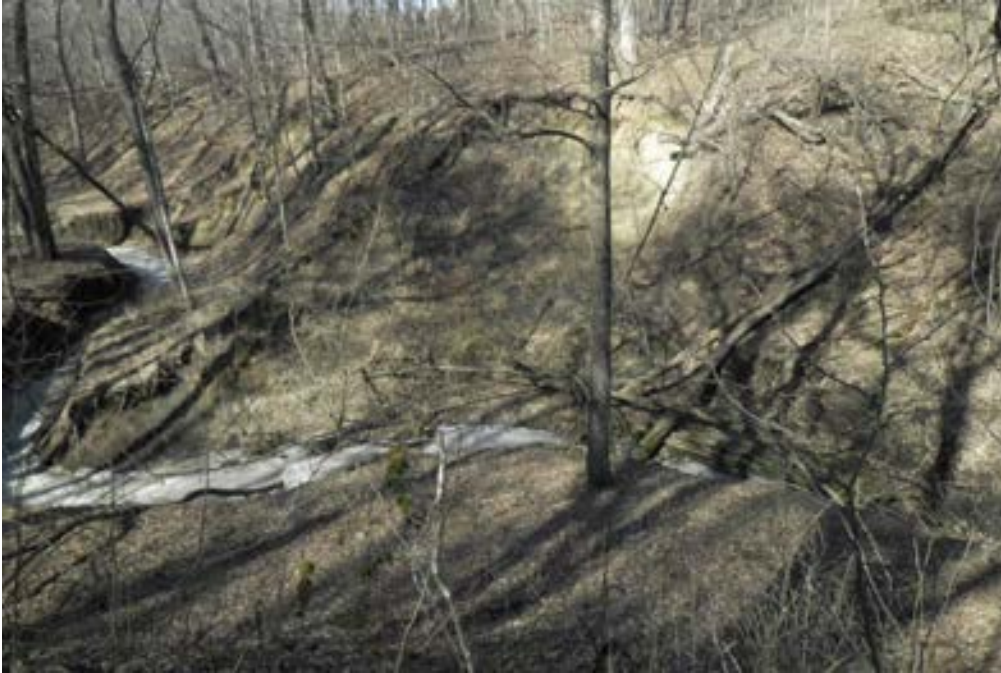
Photo 13. Reach E2. Scarp erosion in right overbank
