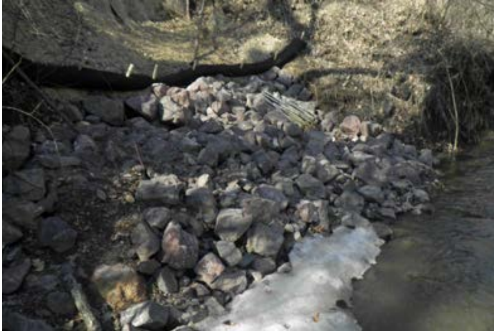
Photo 19. Reach E3. Recently stabilized storm sewer outfall in right overbank
