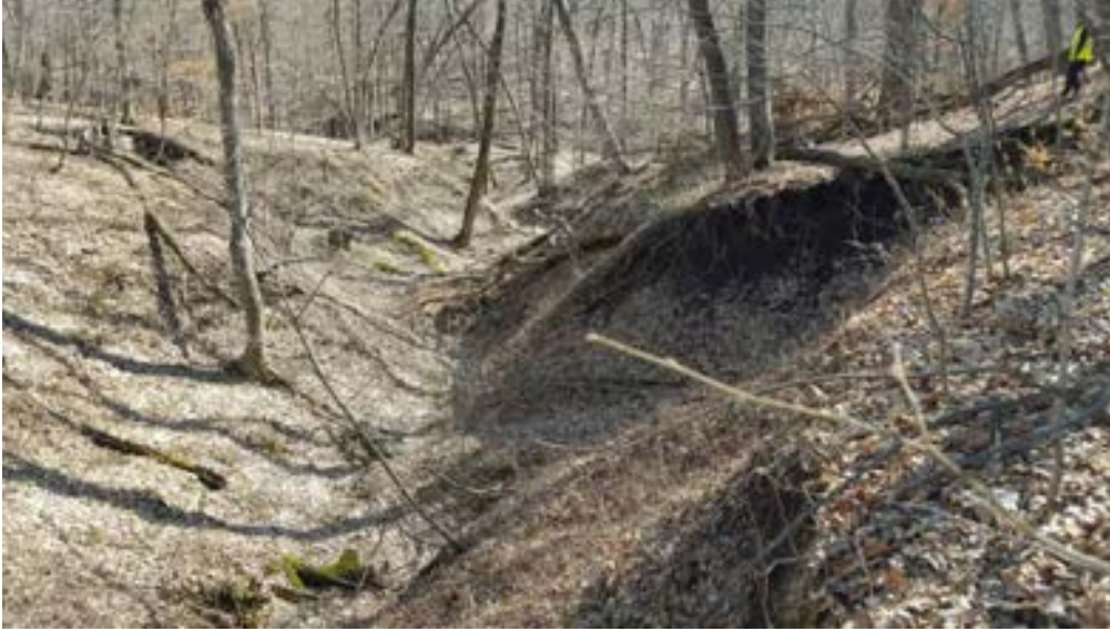
Photo 1. Site D3. Ravine, large scarp on right side of photo (photo is looking downstream)
