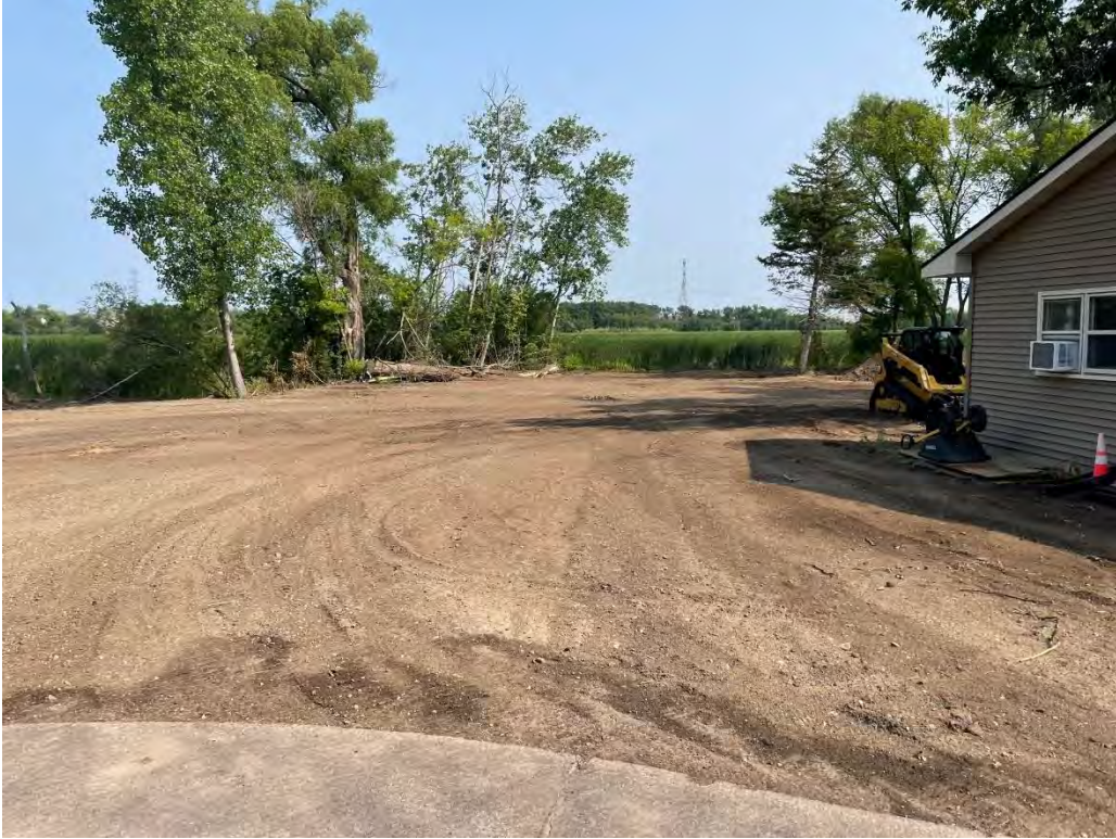
Photo 3: grading and wetland fill area at 5250 Eagle Creek Blvd, Shakopee
