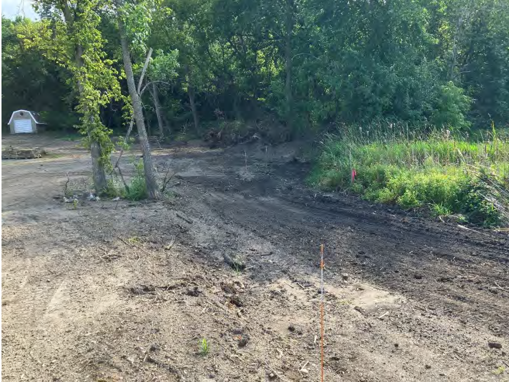
Photo 5: fill removal at 5250 Eagle Creek Blvd, Shakopee
