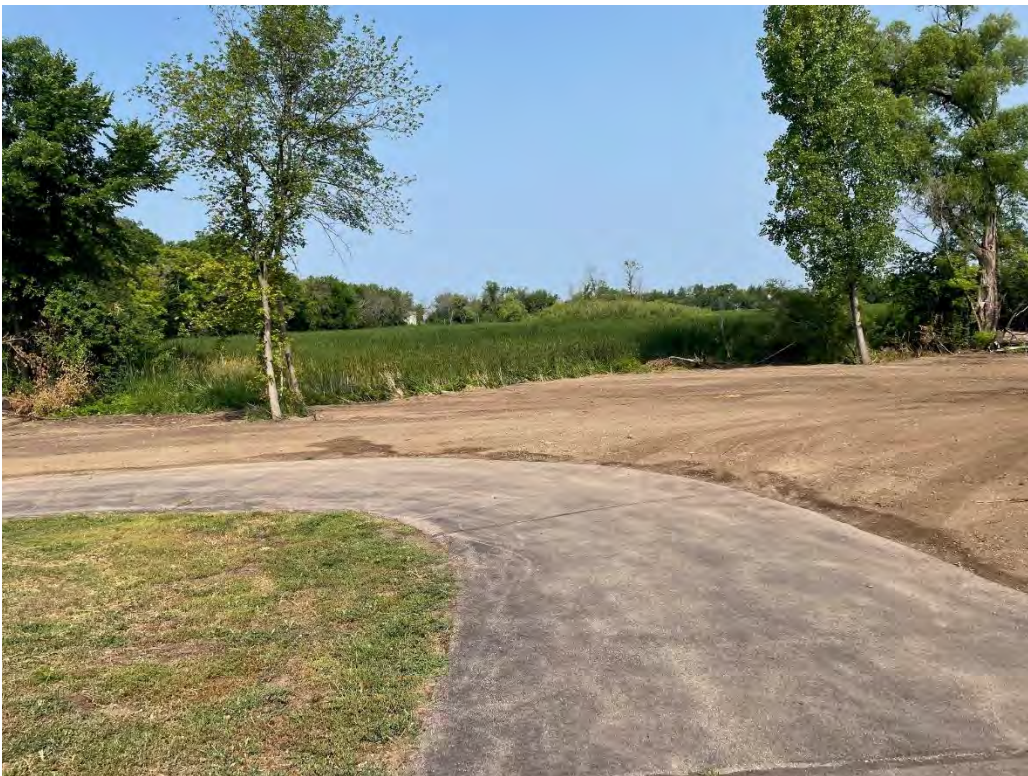
Photo 4: grading and wetland fill area at 5250 Eagle Creek Blvd, Shakopee
